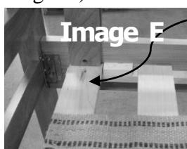
Predrilled hole on Guard Fence
